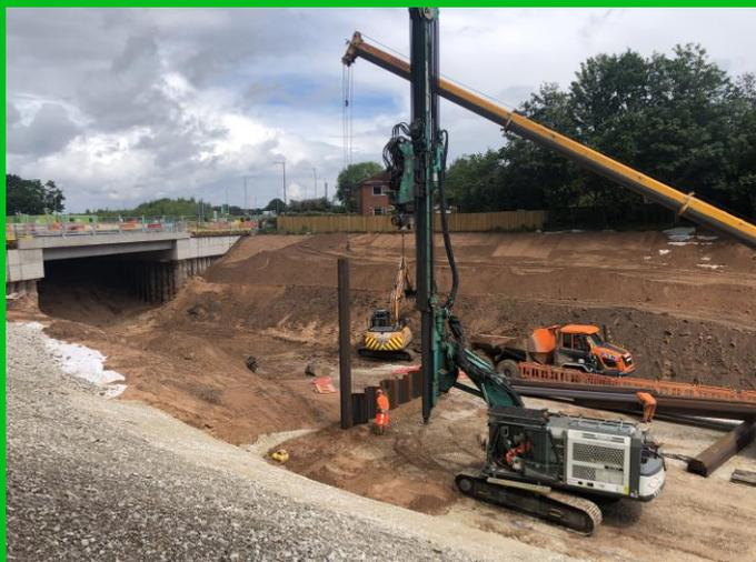
The works included the installation of 186 sheet piles to a depth of up to 10m, using a piling rig and hydraulic vibro-hammer machine. The piling machine transfers vertical vibrations to the sheet pile via a hydraulic clamp, loosening the soil and aiding the installation of piles. The team took the decision to pre-auger and excavate 6m into the ground ahead of the sheet pile installation, in order to minimise the vibration levels on our neighbours.
