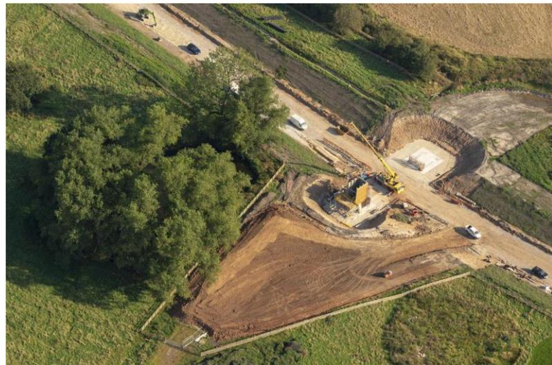
The steel shuttering has been craned into place ahead of 210 cubic meters of concrete being poured during October to form the abutments. The concrete pour will mark the largest pour on the scheme to date.
